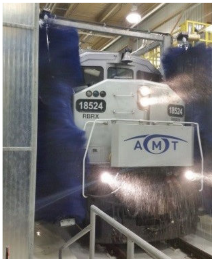
AMT's new maintenance center features an indoor wash facility where trains are washed in five minutes thanks to automated equipment outfitted with giant brushes. Previously, trains were washed outdoors by four employees over eight hours. The new center also reuses 80 percent of the wash water, with the remaining 20 percent treated on site.
