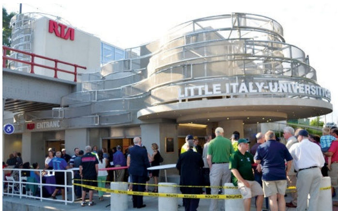
The Little Italy-University Circle Station is RTA's first new Red Line station in 46 years.
