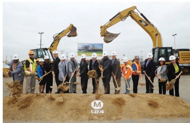
Officials of Los Angeles Metro break ground for the Southwest Yard light rail maintenance and administrative facility.
