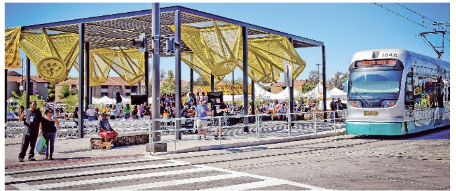
Valley Metro’s extensive public art initiative includes this colorful canopy on its Northwest Extension.
